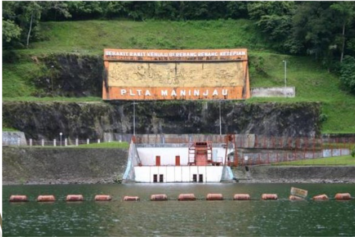
Maninjau Hydroelectric Plant, West Sumatera
