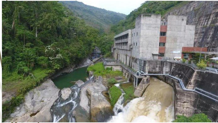
Bakaru Hydroelectric Plant, South Sulawesi
