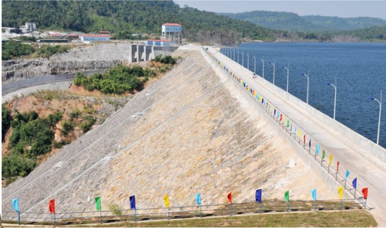
Flags line the Lower Russei Chrum River hydropower dam in Koh Kong province.
